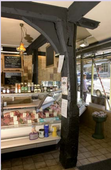
Figure B Evidence of a medieval timber shopfront inside 111 High Street. The modern shopfront is several feet forward, typical of the way many shopfronts have been progressively extended out onto the pavement.
