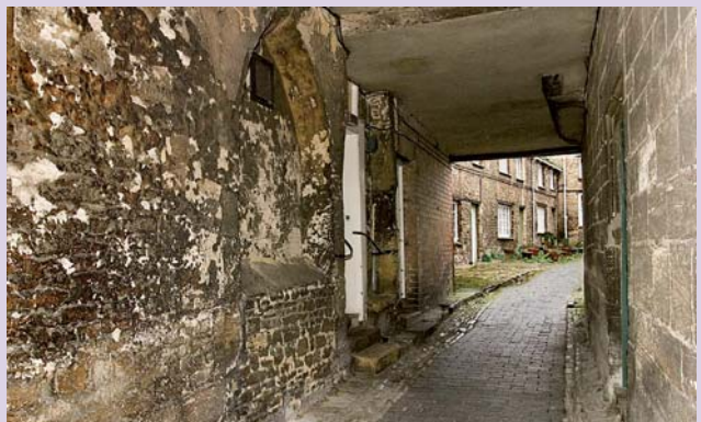
Figure C Blocked 14th-century arches under the carriageway of the George Inn. Possibly they lit small lock-up shops.
