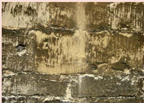
E Coursed, squared and dressed rubble with courses of varying heights; resembling D, but with tool-marks and squared stones in evidence. (Witney Street)
