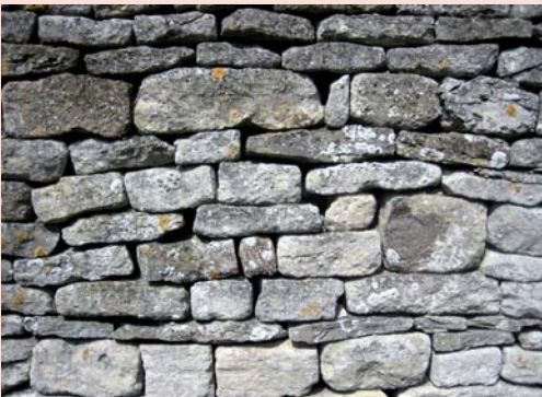
A Semi-drystone walling (Priory Lane): deep joints with no visible mortar, and a mud and clay mix holding the inner stones together.
