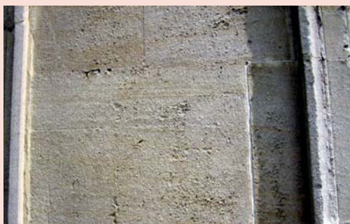
G Coursed and dressed ashlar with fine pointing. This stone is usually only a thin facing on the street front, with rubble behind and in the gable walls.
