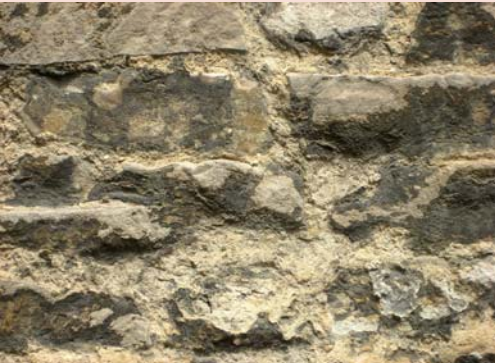
B Uncoursed (randomly arranged) rubble with random-sized stones. (Witney Street)
