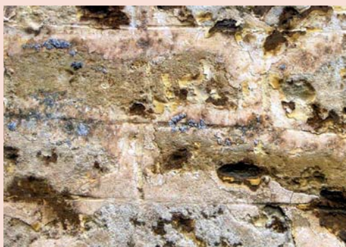
I Scoring in render at 53 Witney Street, creating the illusion of squared ashlar stone.
