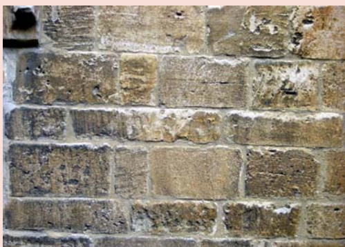
F Coursed and dressed stone of ashlar quality with courses of varying heights; resembling E but with sawn stones in evidence. Pointing may be crude. (Church Lane)
