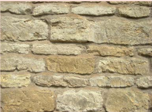
C Coursed rubble with random-sized stones at 33 Witney Street: care has been taken to select similar-size stones and lay them in horizontal lines or courses.
