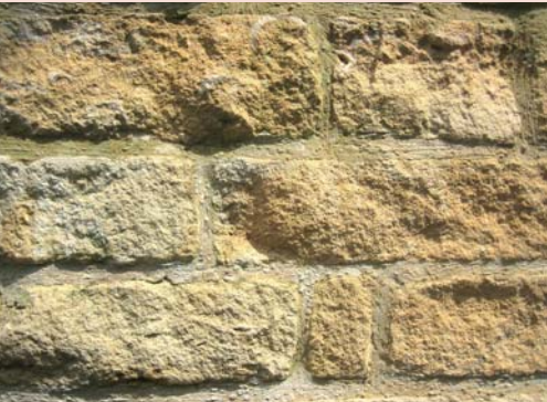
D Coursed and squared rubble with courses of varying heights. This resembles C, but the stones have been squared up and laid in regular courses. (Swan Lane)
