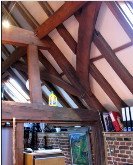
Figure E Part of the roof structure of the hall range, with (right) three carved balls on a corbel in the hall. The balls may represent St Nicholas of Bari, patron saint of wayfarers – appropriate in an inn for travellers by road and river.
