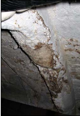
Figure B Chalk vaulting in the cellar under the front range: one of the White Hart's earliest surviving parts.
