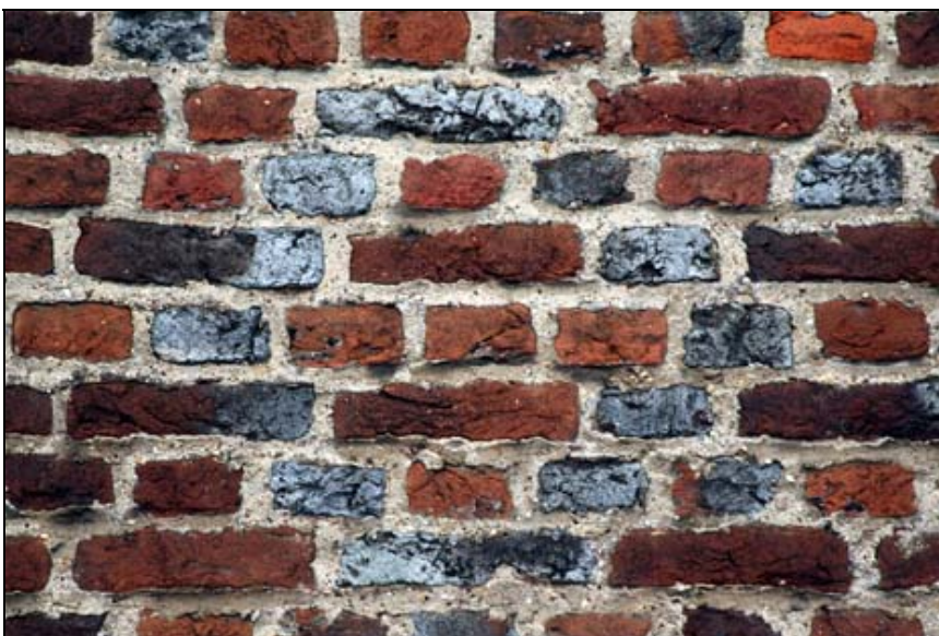
Figure C 1530s brickwork in the west wall, laid in English bond (alternate rows of headers and stretchers), and with a diaper pattern picked out by using over-fired ‘blue’ bricks. This became increasingly fashionable during the 16th century. Though brick later became ubiquitous, this is the earliest that has so far been discovered in Henley. (Photo Derek Toms)
