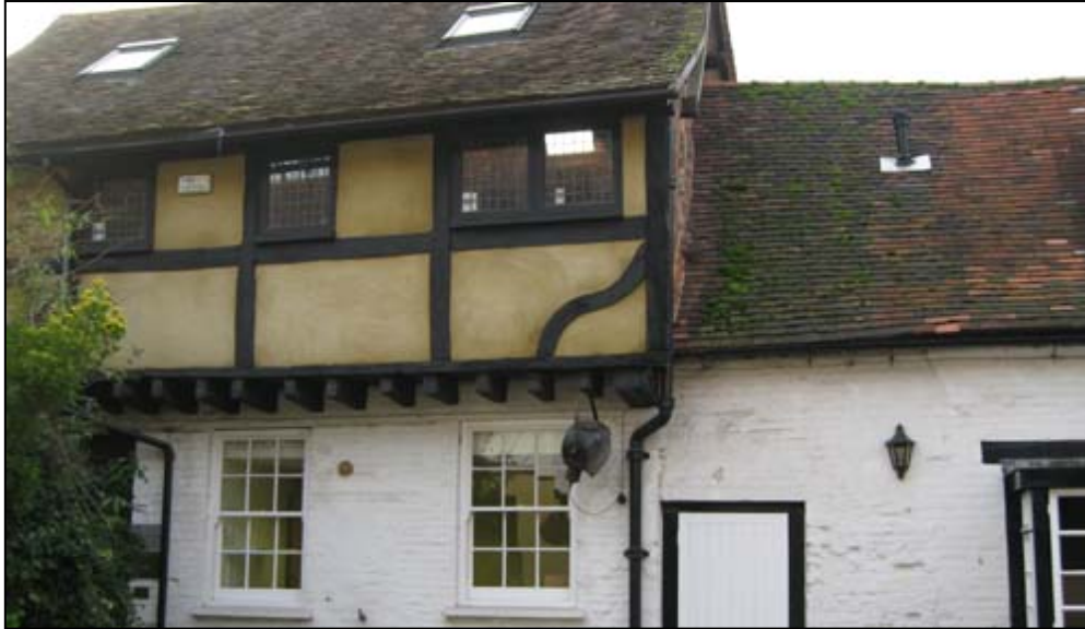
Figure D Part of the former hall on the courtyard's west side, originally open to the roof, and heated by a fireplace in its south wall. The projecting joists may have supported an open gallery, giving access to first-floor chambers further along the range.
