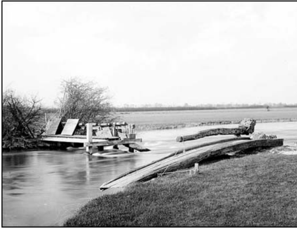
Figure C Eynsham weir and flashlock (upstream from Oxford) in 1883, showing the open passageway next to the weir. The boat-slide (on the right) was a modern innovation, over which light punts could be dragged. (photo: Oxfordshire County Council Photographic Archive)
