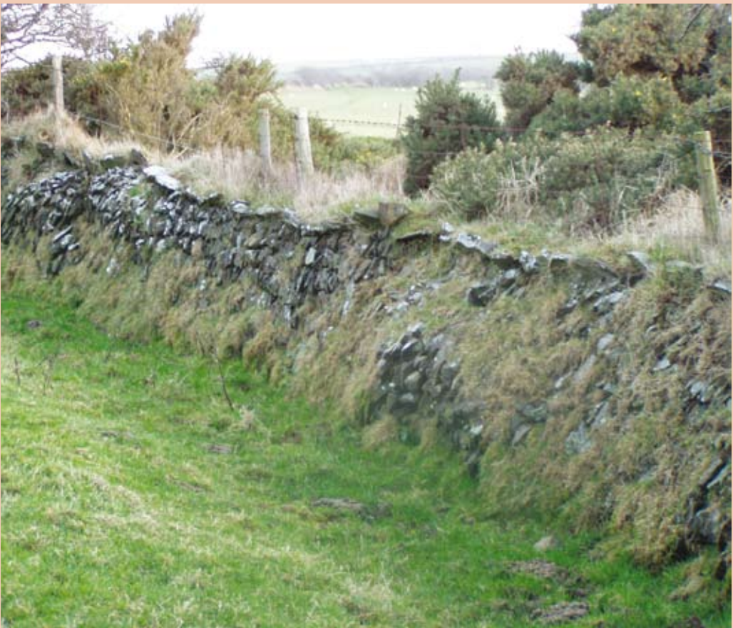
Figure A Corn ditch to keep sheep out of crops on the commons. Temporary fences were raised on low walls of earth and turves and removed when the commons were not in tillage. Later some were stone faced as a permanent barrier. A ditch in front prevent stock jumping over.
