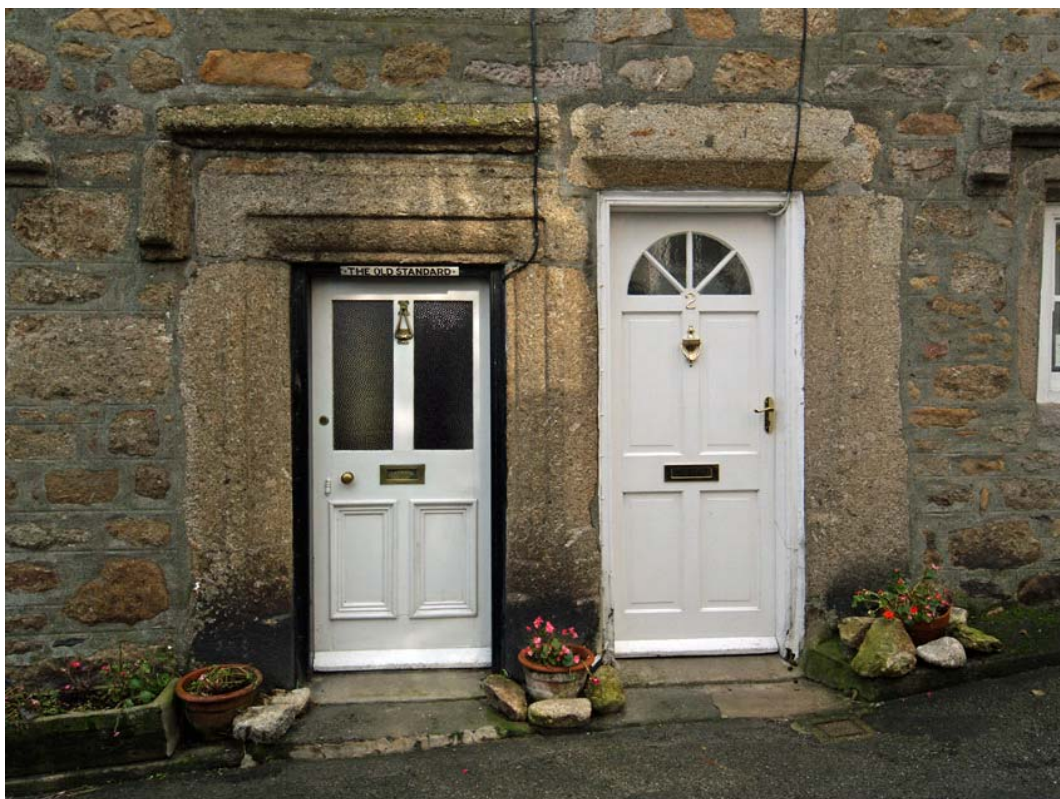
6. The Old Standard: original doorway (left) and later doorway of reused material
