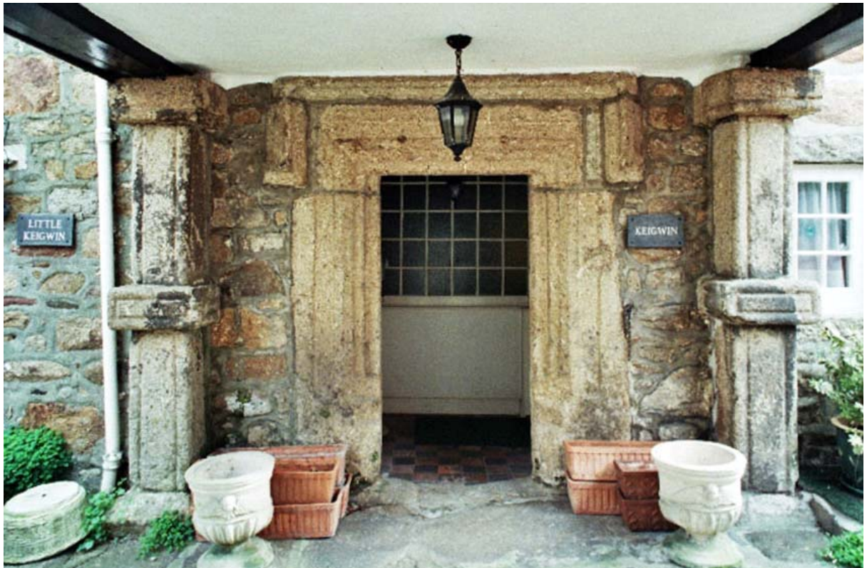
3. Keigwin: moulded granite front doorway and flanking columns of late porch
