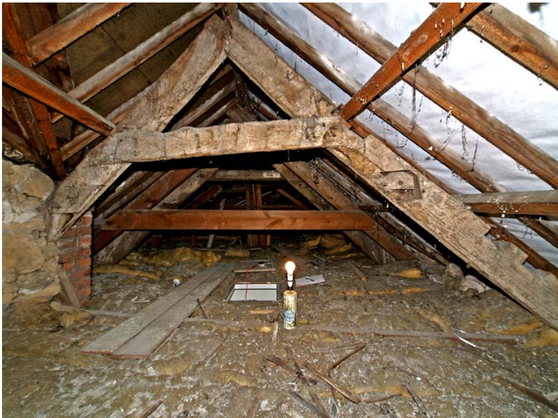
20. Keigwin: roof over east extension to rear range originally with for 2 tiers of collars
