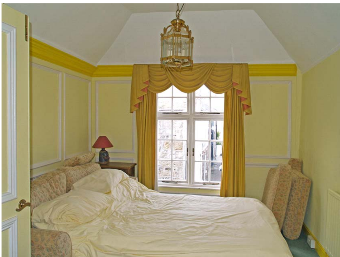
26. Little Keigwin: Bolecion-moulded panelled room over front wing
