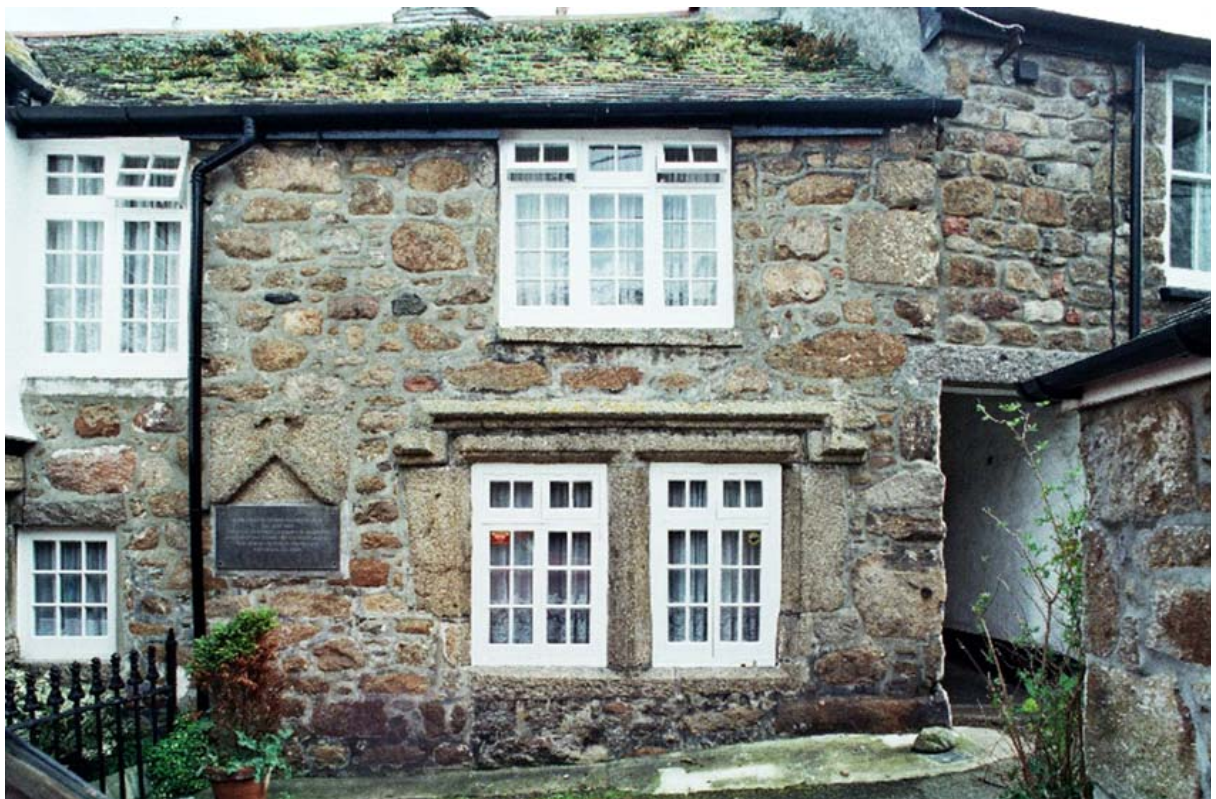
4. Keigwin: restored hall window and reset gable coping of former lateral stack
