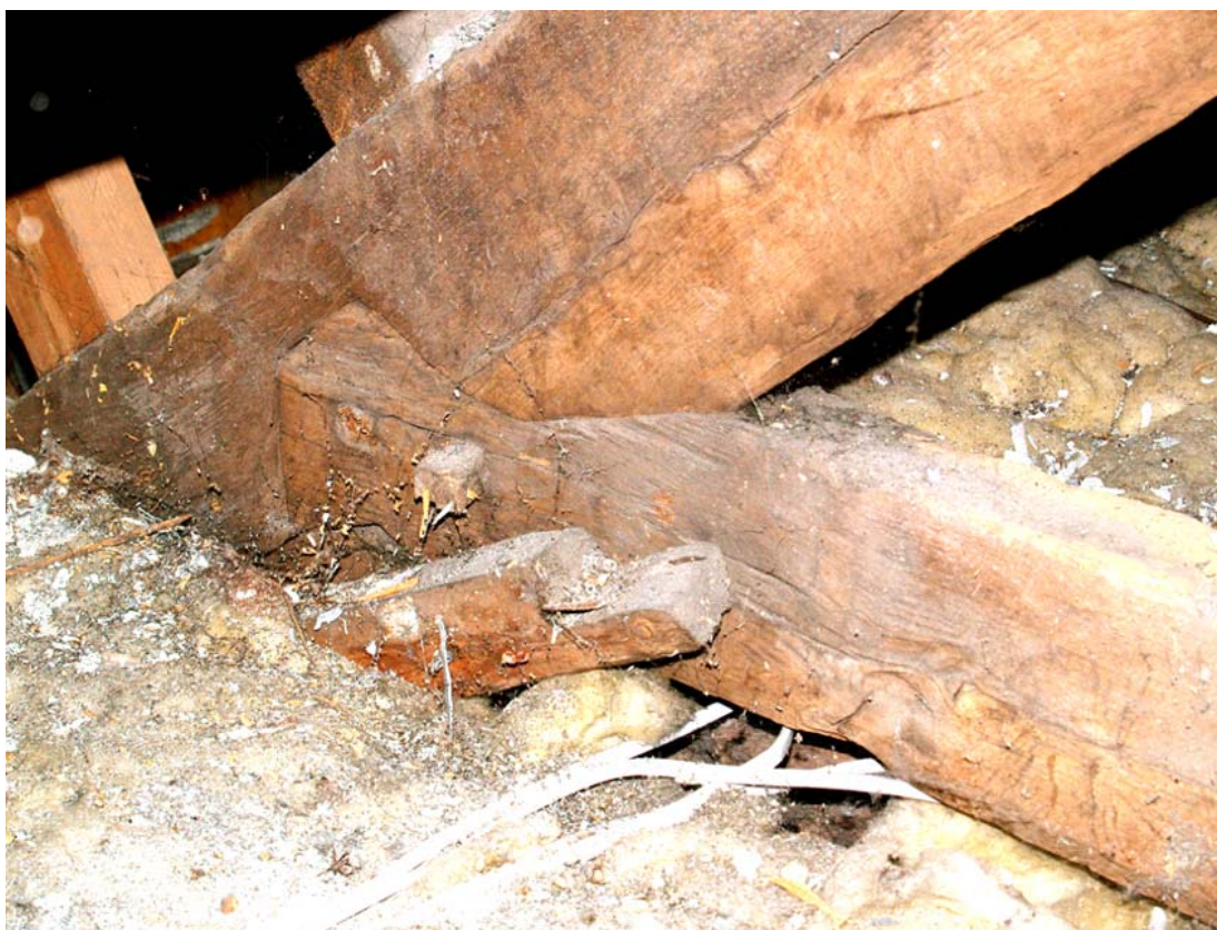
17. Keigwin: front roof structure with detail of collar joint and evidence for former barrel ceiling
