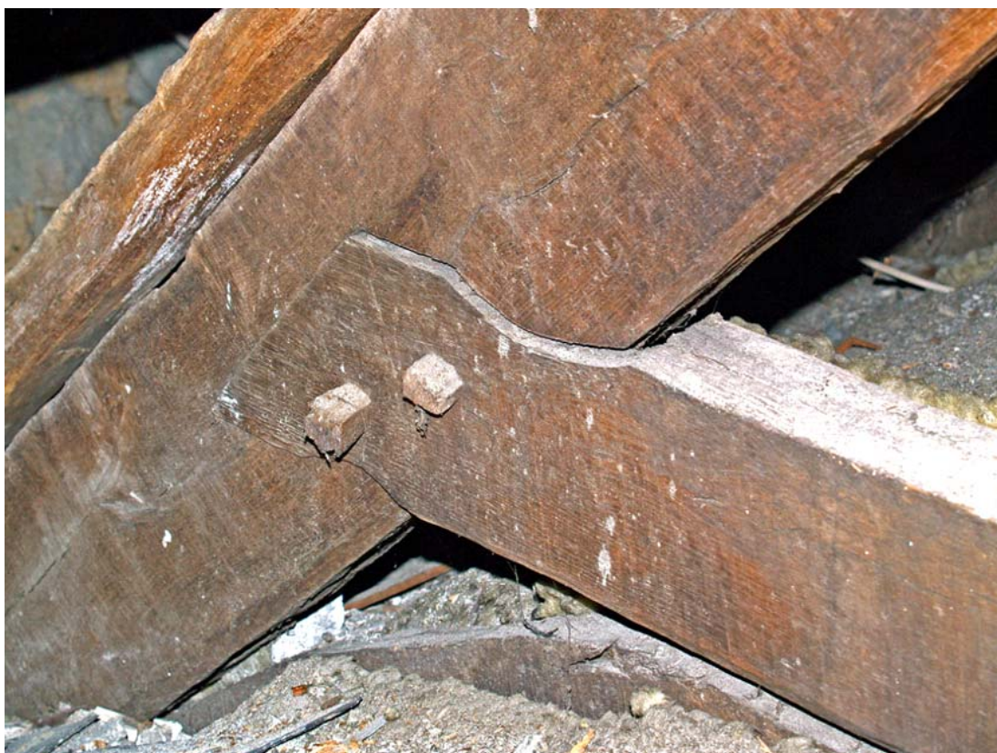
21. Little Keigwin: front roof structure detail of collar joint and brace supporting barrel ceiling
