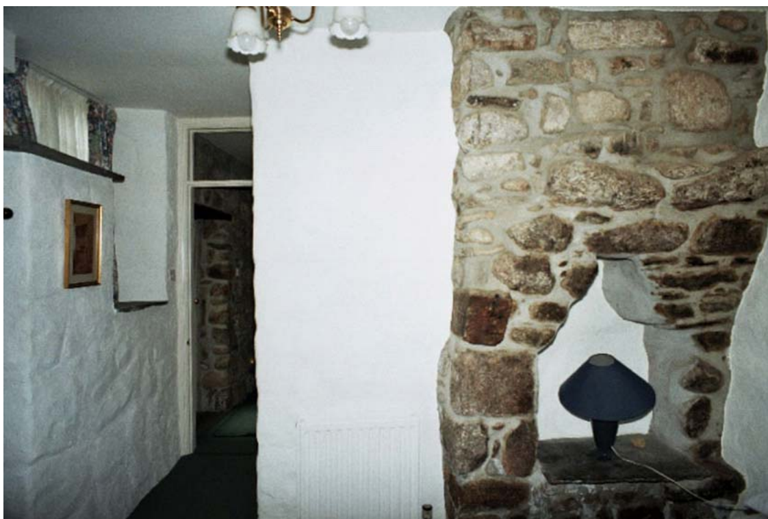
28. Little Keigwin: 18 th century oven inserted to 17 th century fireplace since mostly removed
