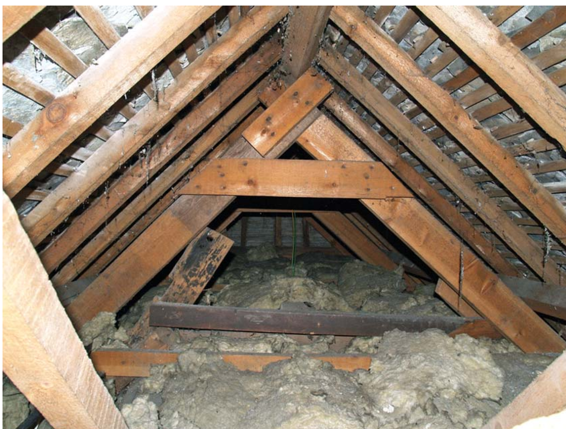
21. Little Keigwin: front roof structure detail of collar joint and brace supporting barrel ceiling
