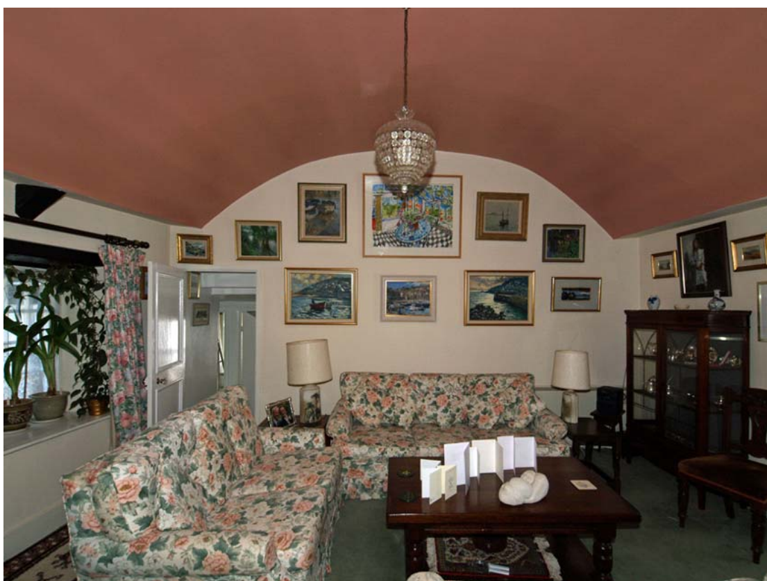
16. Keigwin: chamber over parlour with plaster barrel ceiling and 2-panel door
