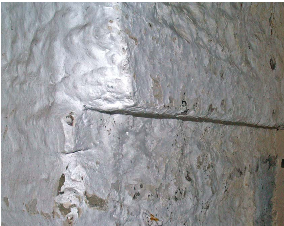
34. Old Standard: corbelled beam shelf for pilchard-pressing floor
