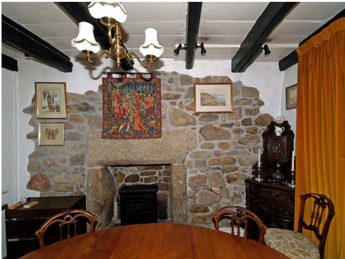
14. Keigwin: original parlour fireplace and ceiling with original chamfered joists
