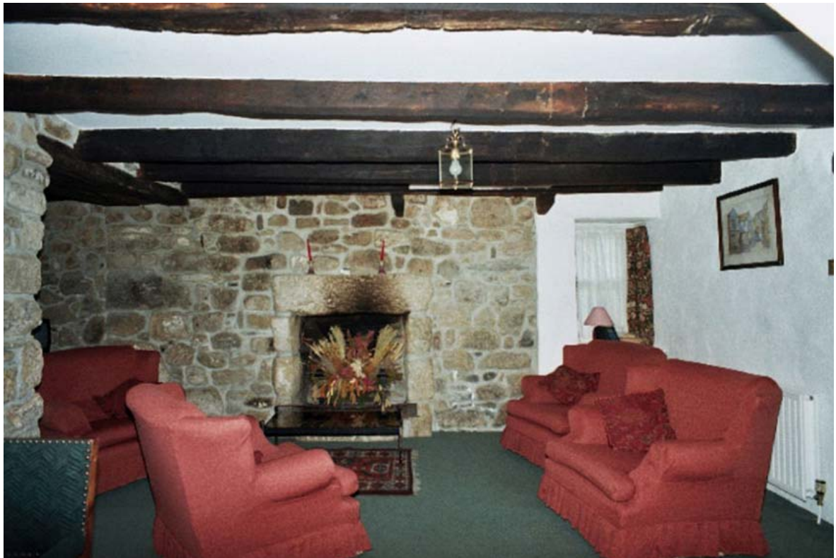
23. Little Keigwin: main front room with later inserted fireplace (note chamfered joists)
